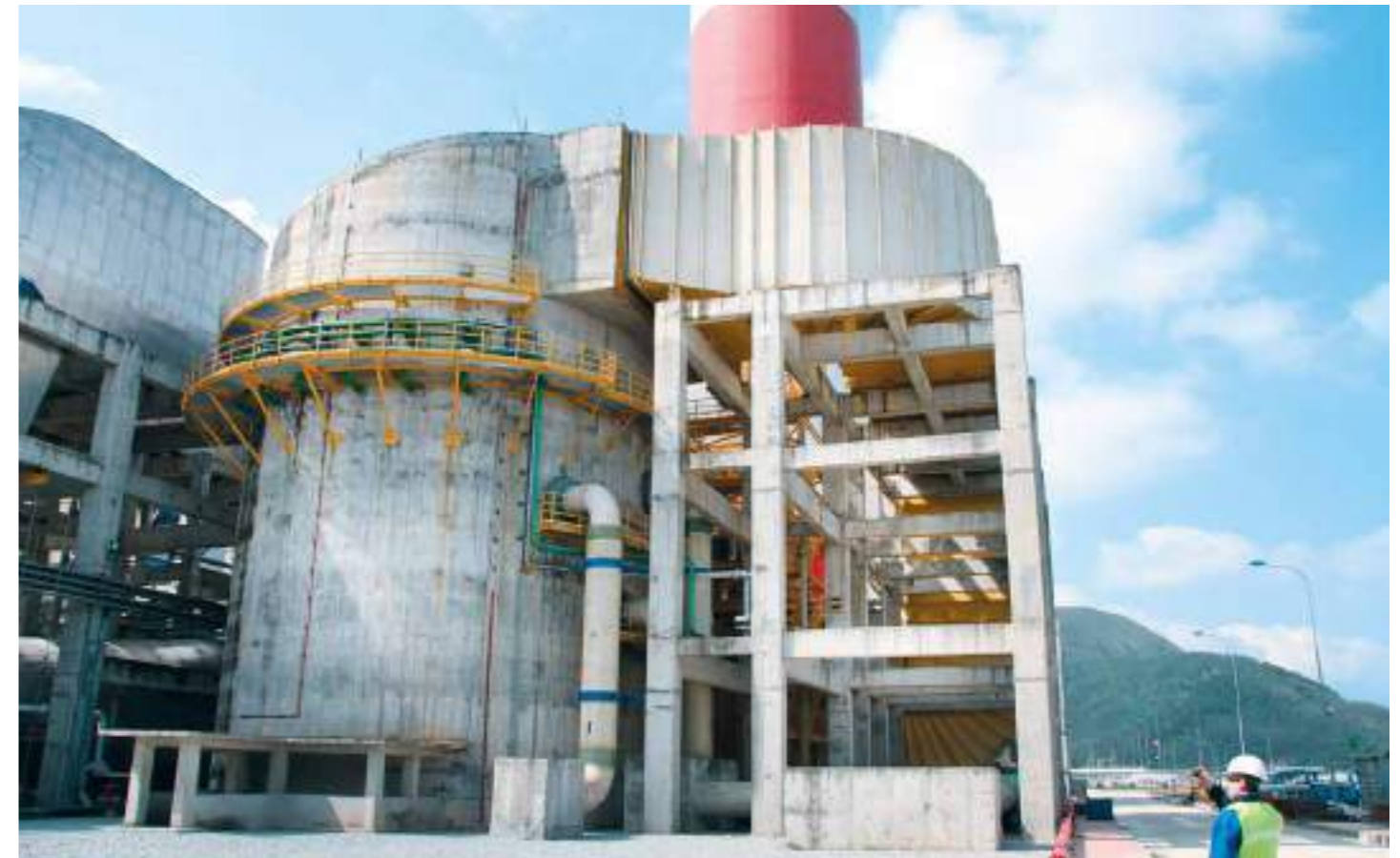
◀ Seawater FGD at Central Power Plant #6, Venezuela ▼ Seawater FGD at Vung Ang power plant, Vietnam
