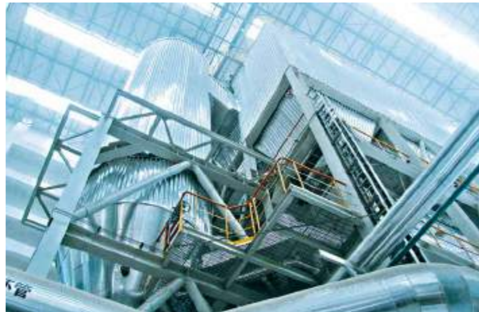
▲ Turbo-CDS (Dry FGD) waste to energy power plant, Haikou, China
