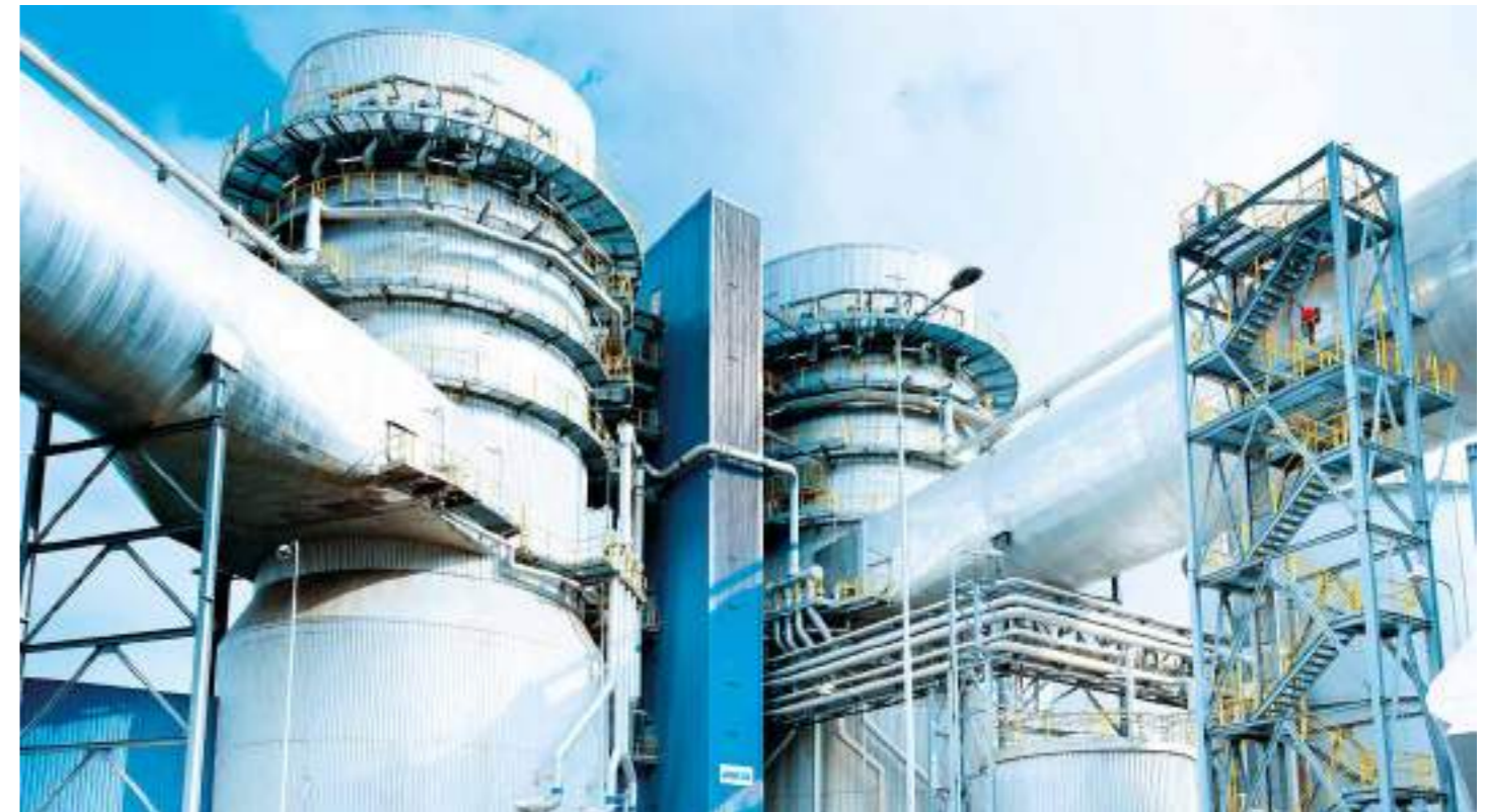
▲ Wet limestone FGD, Tušimice, Czech Republic
