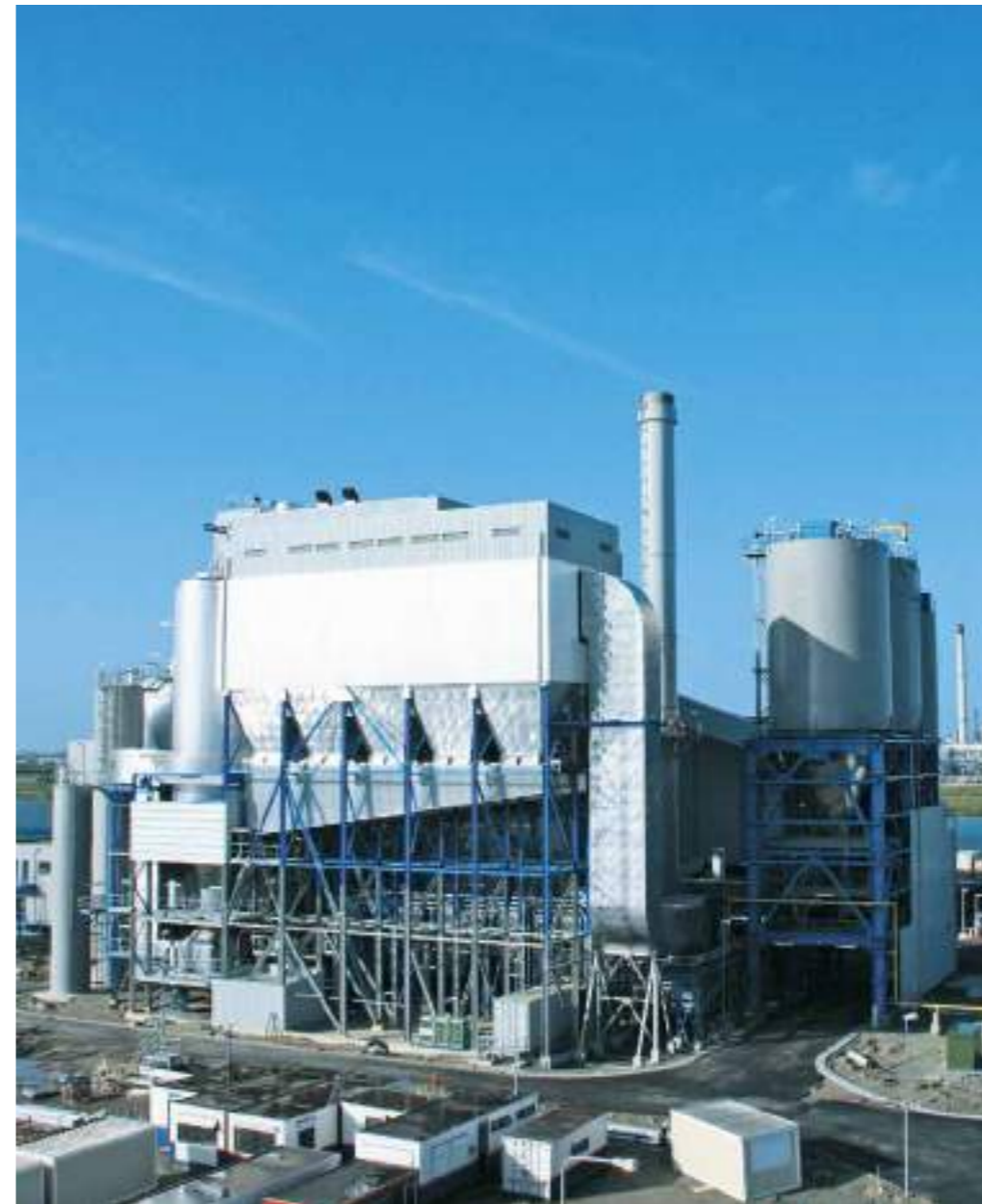
◀ TurboSorp, Fabric Filter, SCR, Moerdijk, Netherlands
