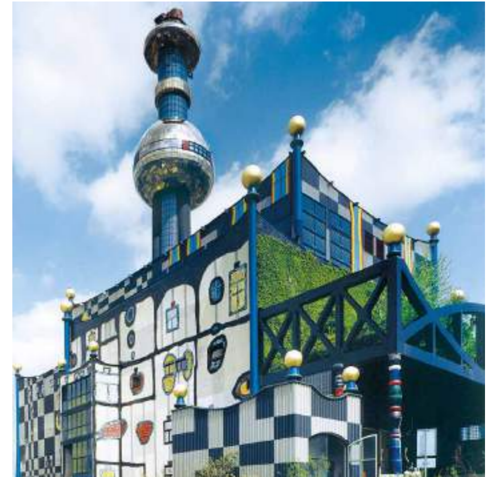
▲ Wet scrubber, tail-end SCR, two trains, Spittelau, Austria
